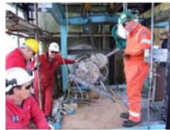
Installing iNPIPE's Plugging System
